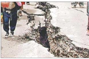
FIGURE 2. DAMAGE DUE TO EARTHQUAKE 1991 (A) COLLAPSE OF HOUSES AT UTTARKASHI, (B) CRACK IN THE HOUSE AT CHADETHI, (C) SLUMPING OF BHATWARI MARKET, (D) CRACKS IN BHATWARI ROAD
