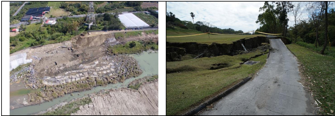
Photo 2 Damage building and infrastructures induced by liquefaction around Tainan City area (Photo: Tainan City Government)
